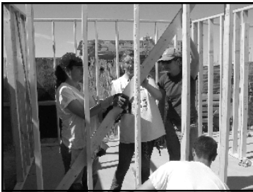
Holding up the frame
